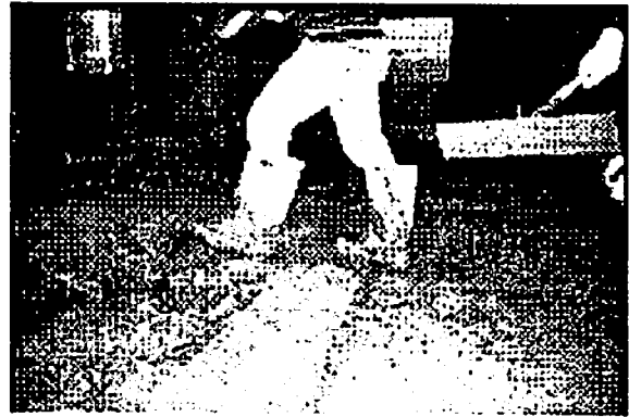
Mat is nailed down and concrete is poured directly over top.
