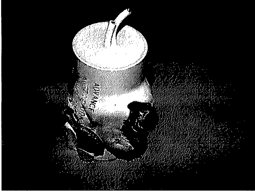
Picture 2. Typical blown capacitor
