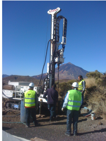
Figure 13. Drilling of one of the boreholes devoted to study the transport of radon under different geological settings.
