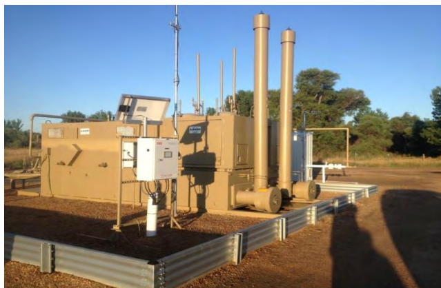
Figure (3): A typical three-phase separator station. Here, the oil, gas and water are separated.
