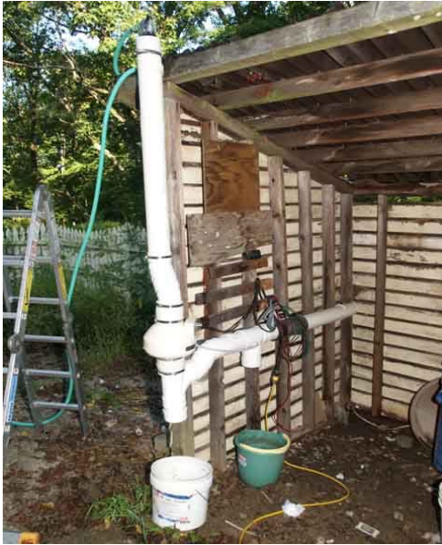
Photo 6 – Drainage test setup
