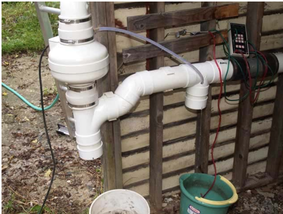
Photo 10 – HP190 by-pass drain test
