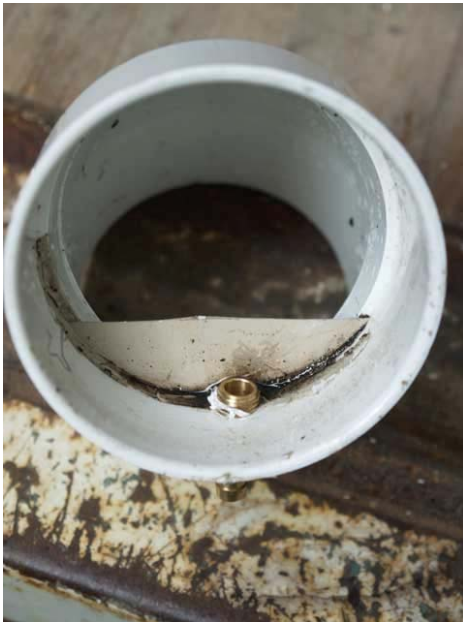
Photo 3 - Dilts water dam
