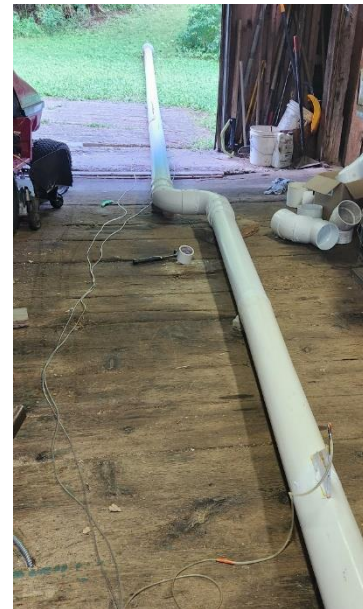
Figure (29): Six-inch 90 degree sweep offset fittings
