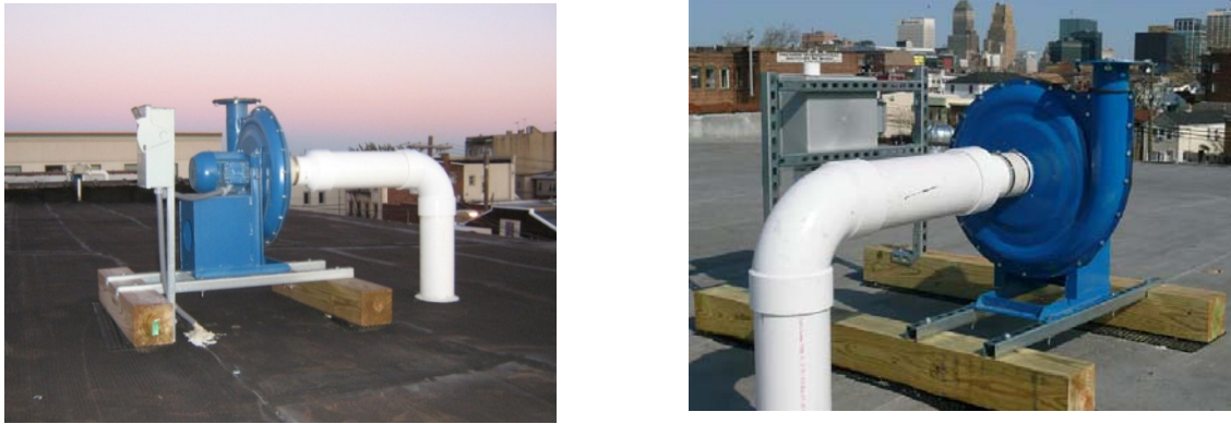
Figure 5: FTF 40/75 Installed on the Roof
