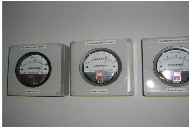
Figure 7: System Vacuum Gauges
