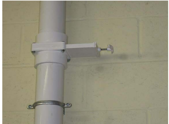
Figure 9: Slide Gate Damper
