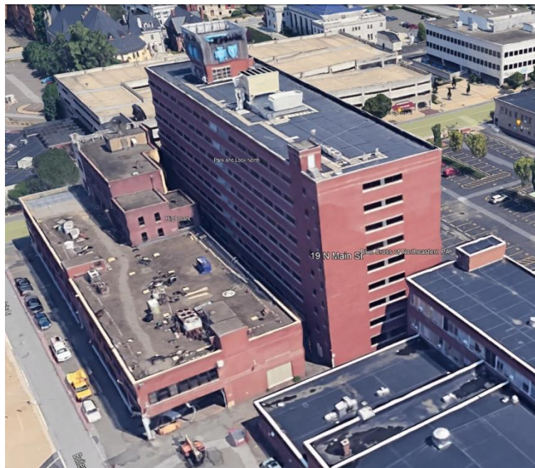
Figure (19): 10 story building requiring a radon mitigation system design
