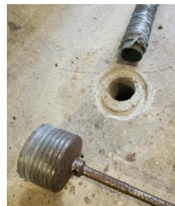
Figure (14): 2.5" core enlarged to 5" core
