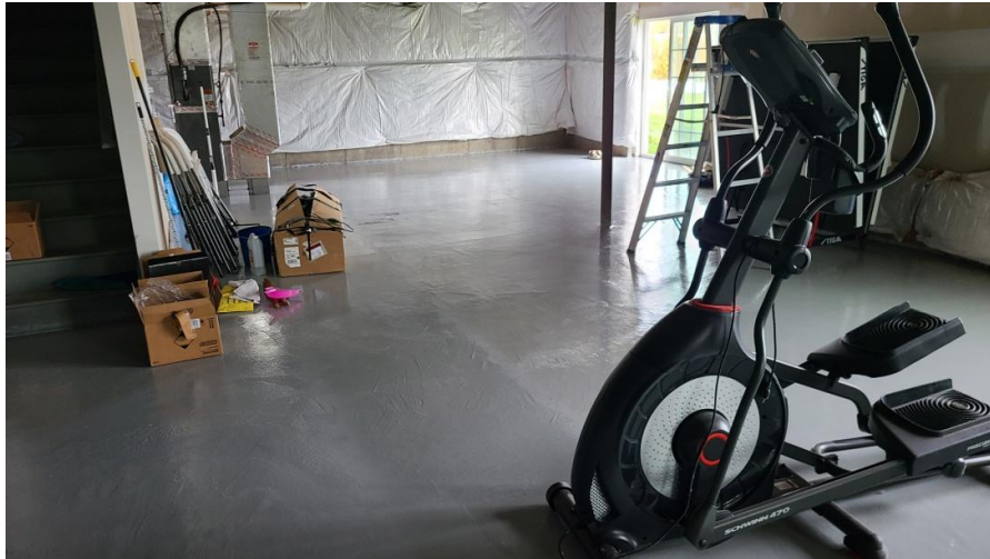
Figure (11): Study house walk out basement with epoxy painted slab
