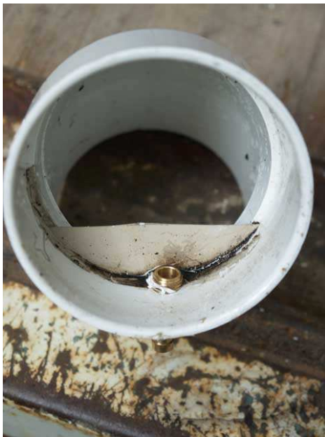
Photo 3 - Dilts water dam
