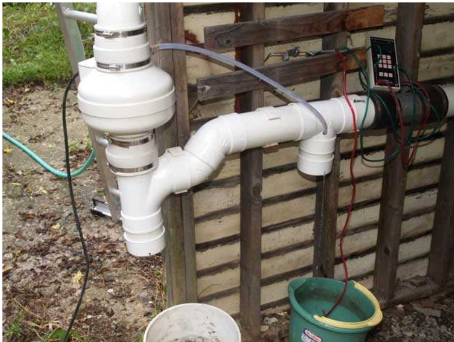
Photo 10 – HP190 by-pass drain test
