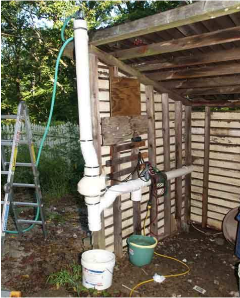
Photo 6 – Drainage test setup
