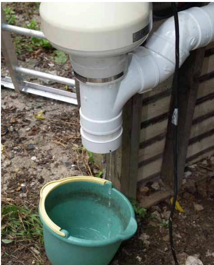
Photo 8 – Drain hole test
