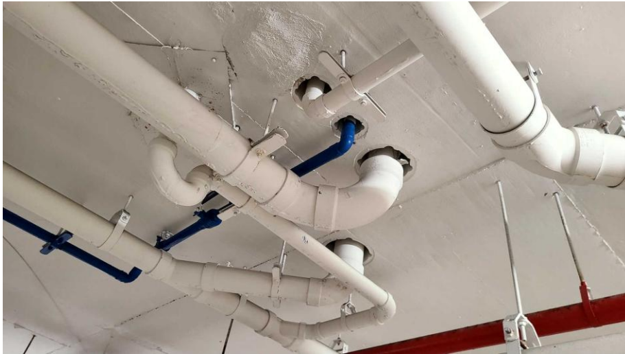
Figure (5): Plumbing openings in ceiling of garage
