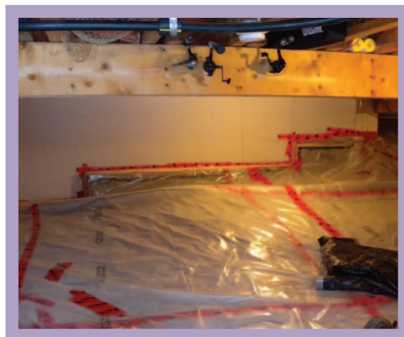
Photo 6 – Membrane and Wall Attachment
