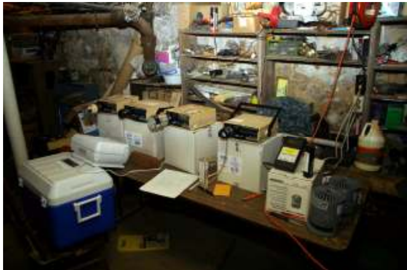
Figure 5 – Portable HEPA filter in front of WL-617
