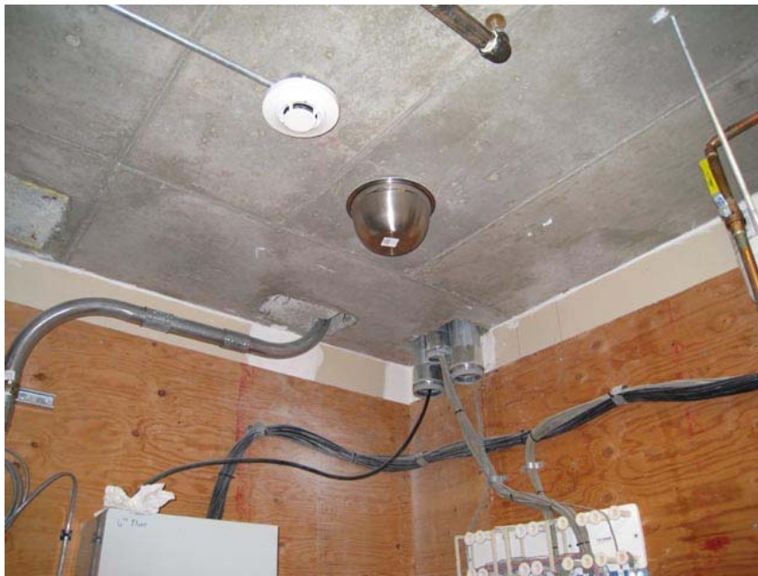
Figure 5 E-PERM Emanation of ceiling of electrical room
