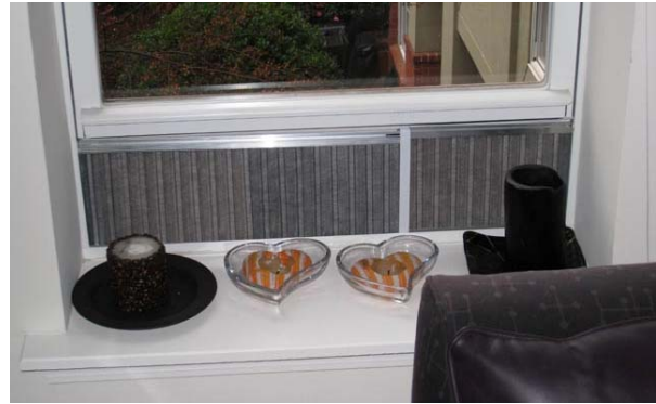
Figure 9 Occupant placed screen in window opening for ventilation
