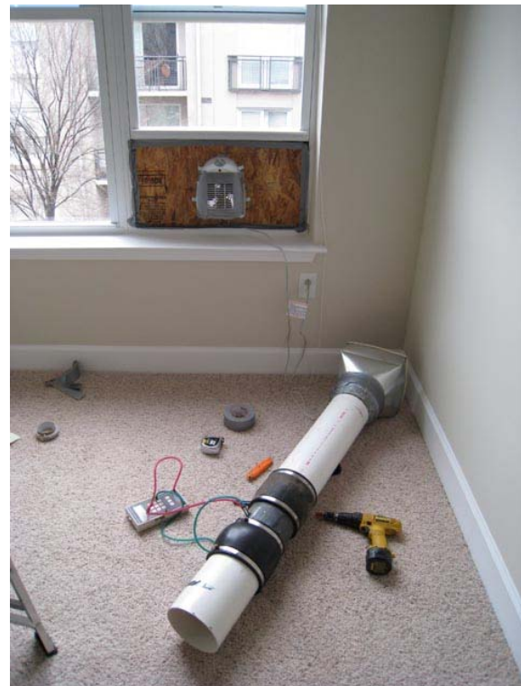
Figure 10 Combination ventilation fan and heater with calibrated flow grid airflow measuring setup
