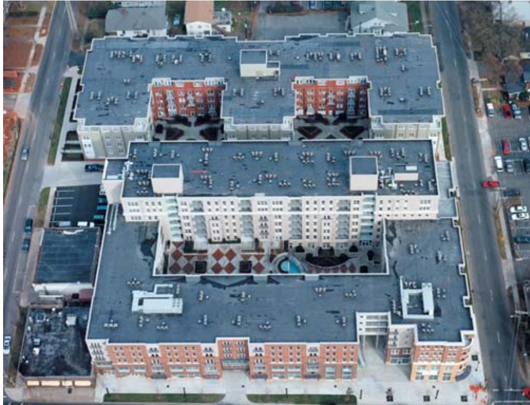
Figure 1 Aerial Photo of both Buildings
